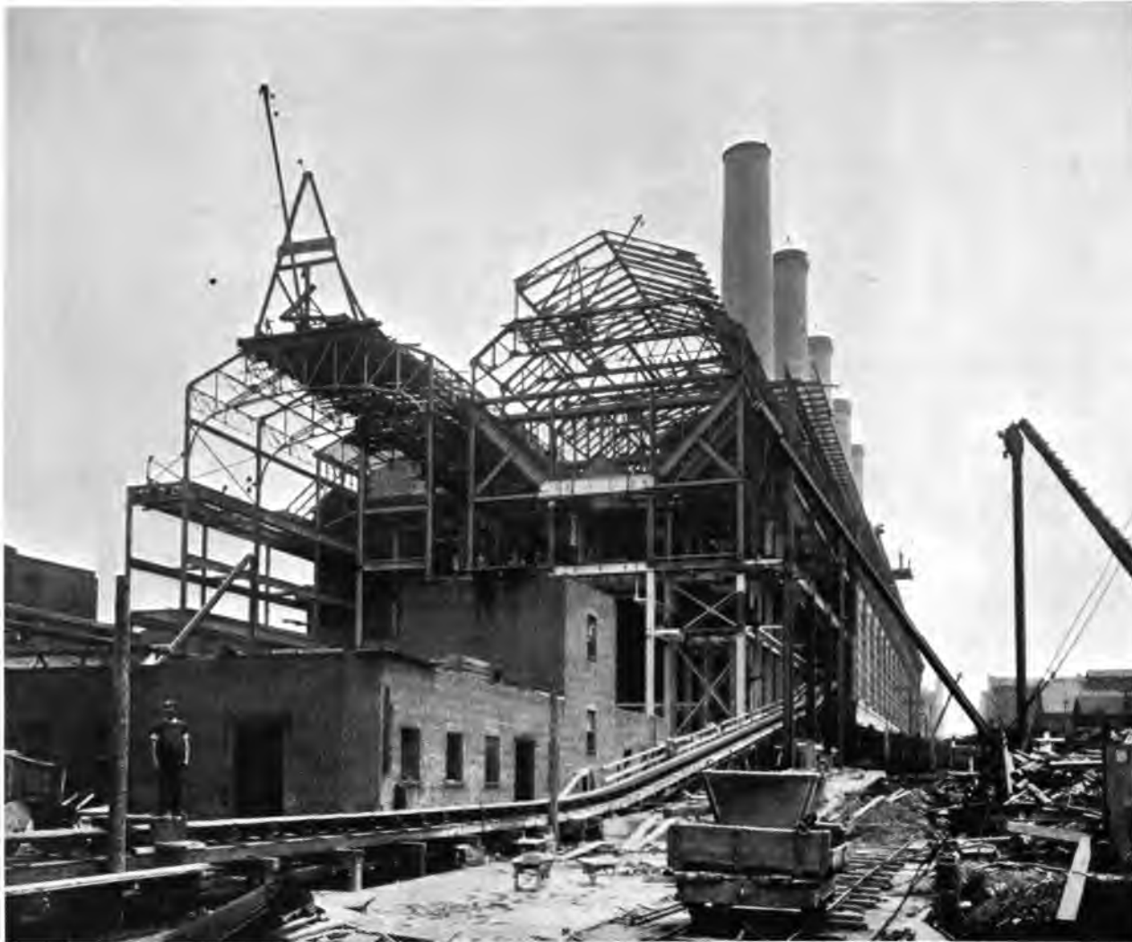
WEST END POWER HOUSE IN COURSE OF ERECTION
